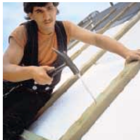
Fig. 6: Nailing the bearing battens
