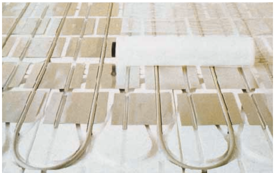
Fig. 22: Floor heating
