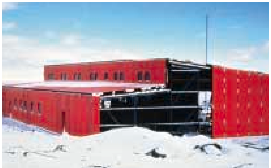
Fig. 20: Australian research center in the Antarctic. The building consists of 100 mm to 150 mm thick Styropor sandwich units which have to withstand temperatures down to 40 °C (-40 °F) and wind speeds of up to 280 km/h (174 miles/h).
