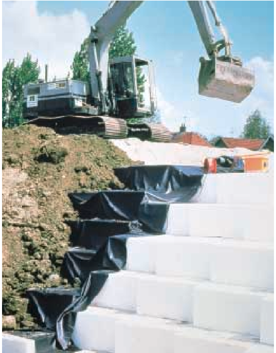
Fig. 28: Styropor as a load-distributing substructure
