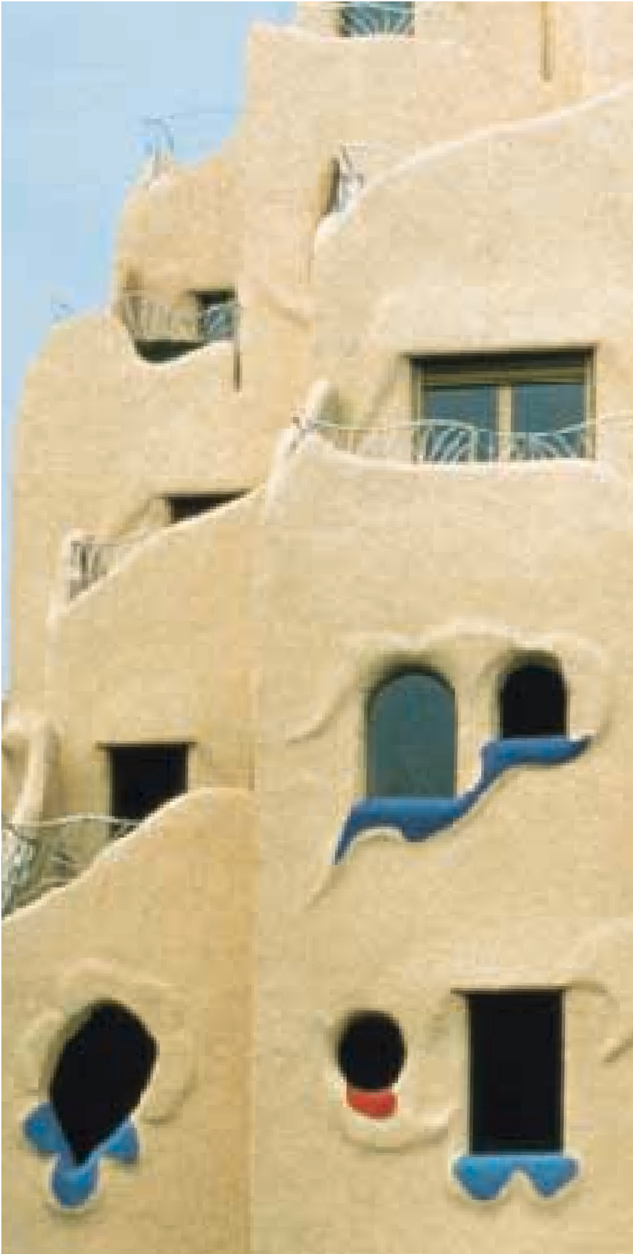
Fig. 15: Insulating plaster facade Building: Les Grottes, Geneva
