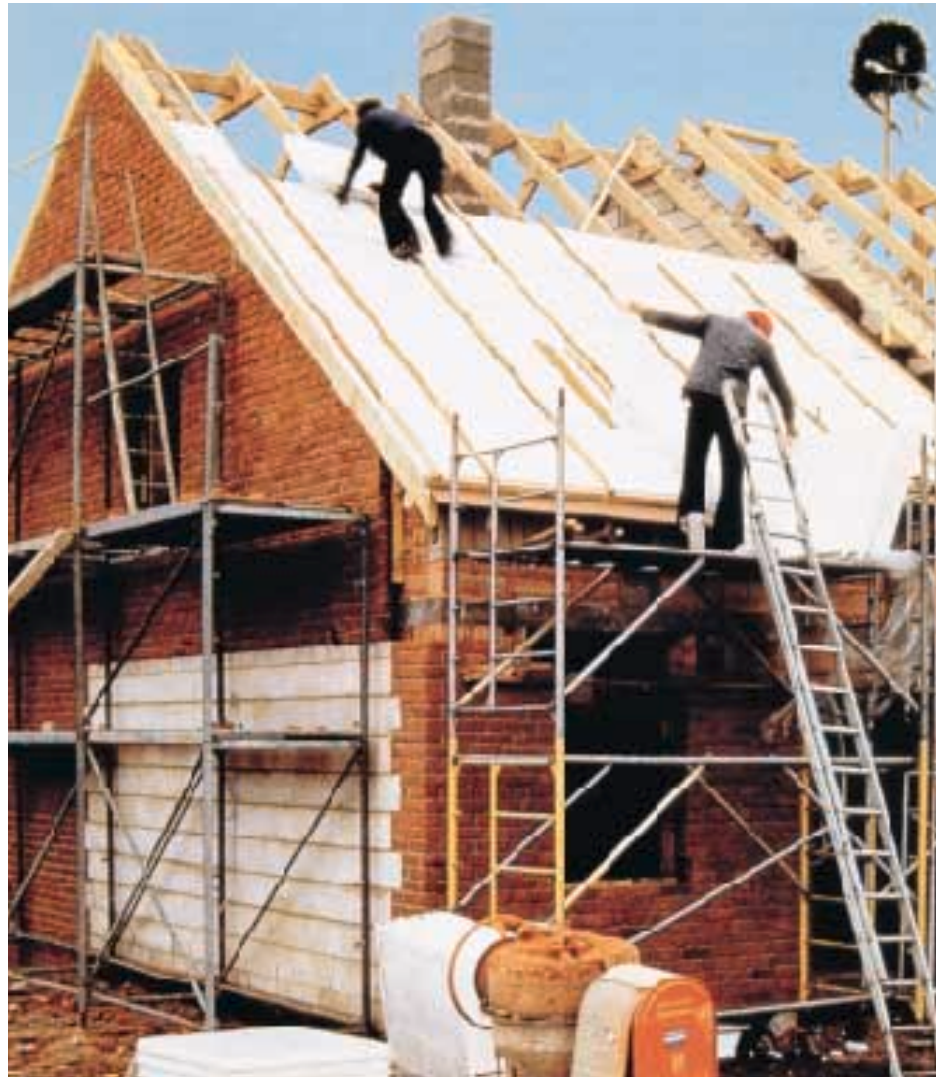
Fig. 4: Construction and insulation with Styropor rigid foam
