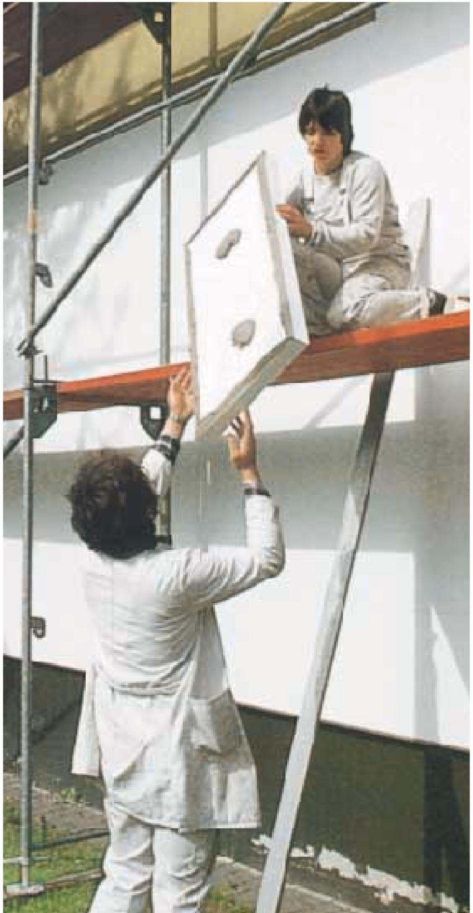
The production of lightweight large-panel wall units with a plastercoated external insulation is particularly widespread in the USA. The supporting board is mounted on a sectional steel frame and provided with the insulation and fabric-reinforced plaster coating (Fig. 10). The easy-to-assemble compound units give the impression of a solid external wall.
