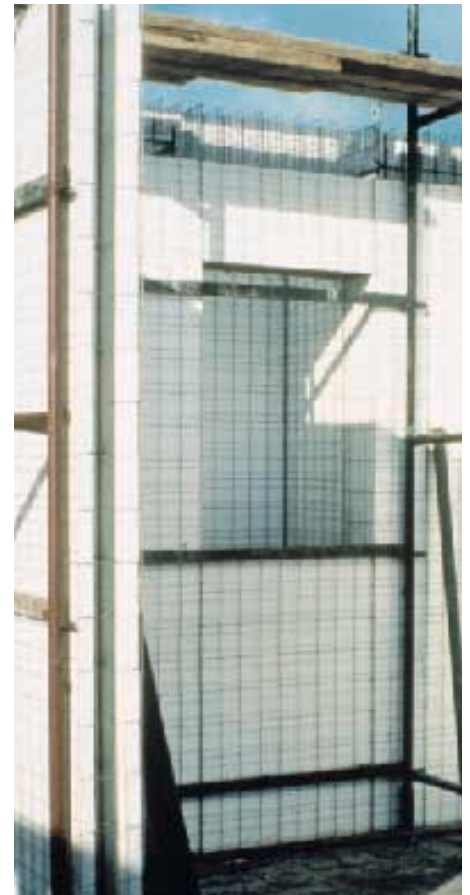
Fig. 26: Wall formwork system
