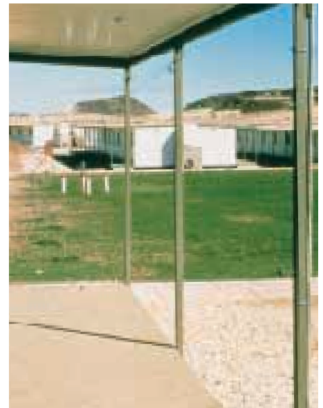
Fig. 19: This region in West Australia suffers from cyclones and summer temperatures of 45 °C (113 °F). All the buildings of this settlement were constructed using the Styropor sandwich technique. The 50 mm to 75 mm thick sheet steelcoated panels were brought 1600 km for this project.
