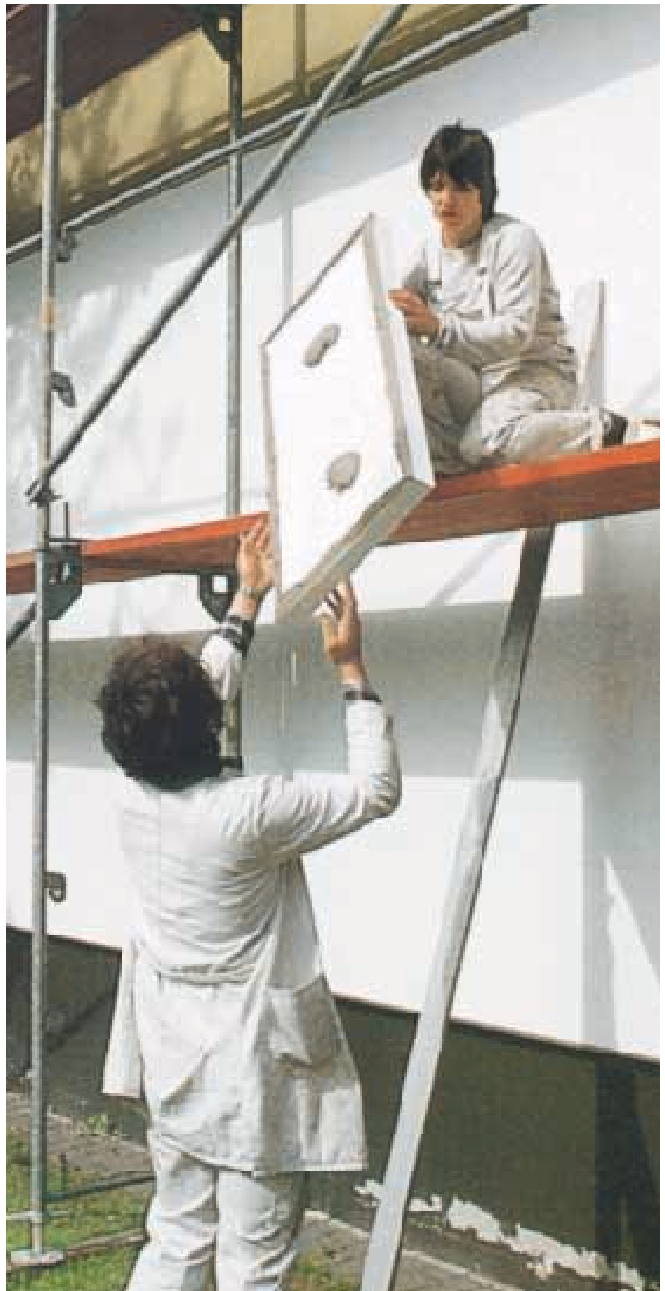
Figs. 8 and 9: External wall insulation with the composite thermal insulation system
