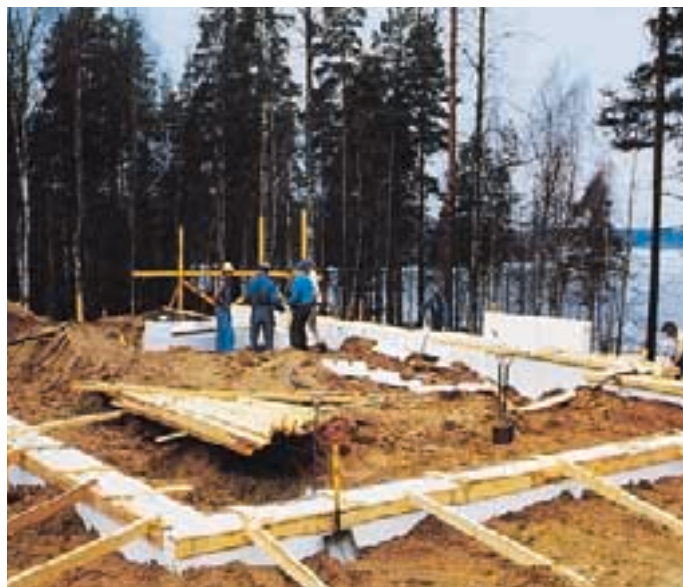
Fig. 28: Styropor as a load-distributing substructure
