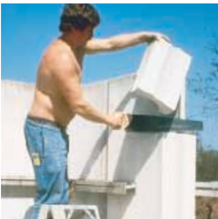
Fig. 16: Styropor concrete wall units
